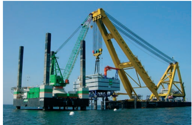
Figure 5.5 Installation of HornsRev transformer
