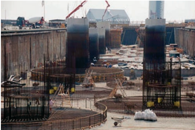
Figure 5.4 Foundation manufacture at Burmeister & Wain shipyard dry dock
